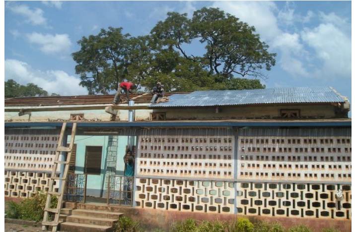
Renovations underway at the mission residence
