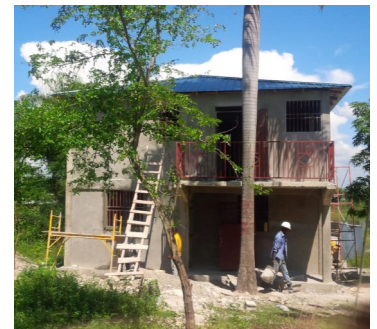
Administrative offices, LaHoye
